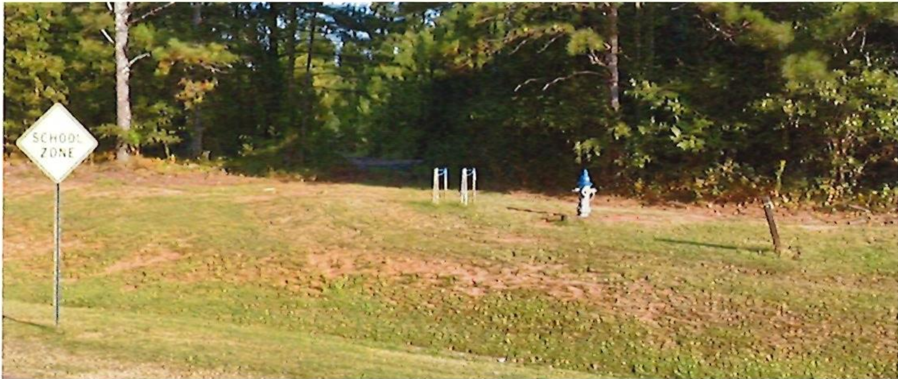
Existing drainage swale, hydrant, and utilities along New High Shoals Road.
