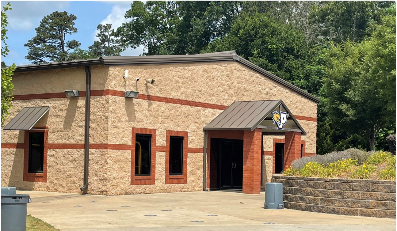
Existing Field House Exterior
