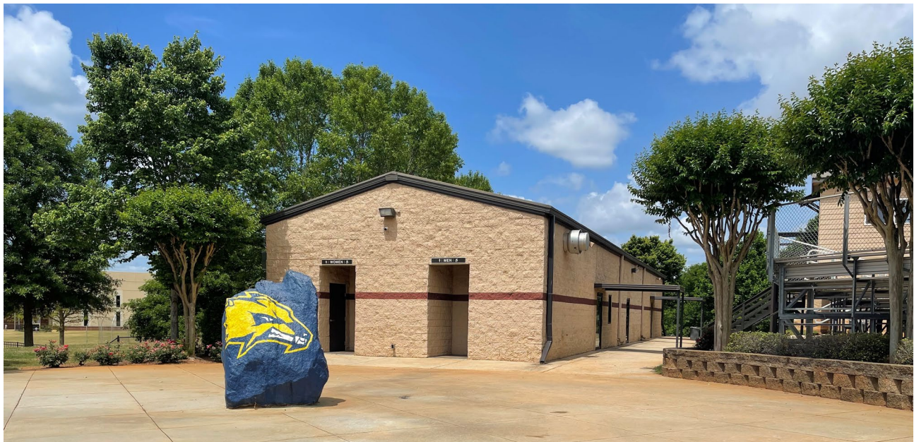
Existing Field House Exterior
