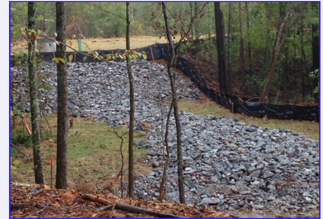
McNutt Creek Trunk Sewer - Soil Erosion Prevention
