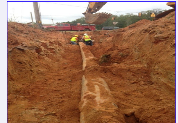
Installation of water main on Mars Hill Road
